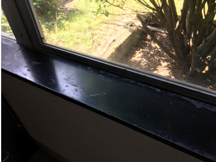
Photograph 5: Area of absent caulking, Burncoat room F2.
