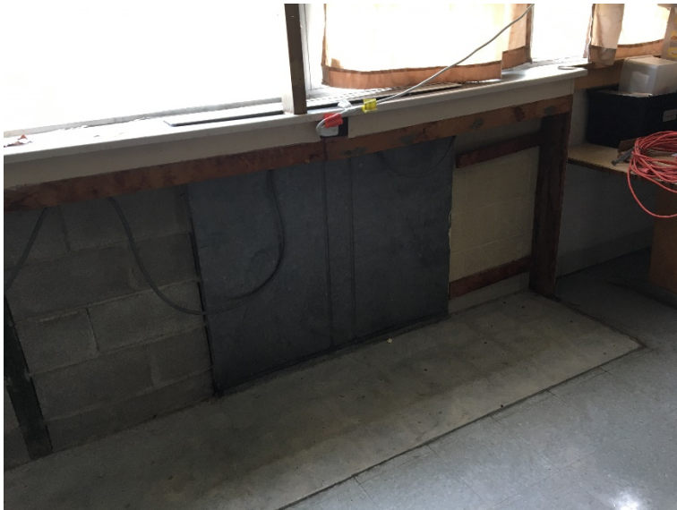
Photograph 4: Counter along window demolished as part of asbestos abatement, showing plenum riser, Burncoat room F-8.
