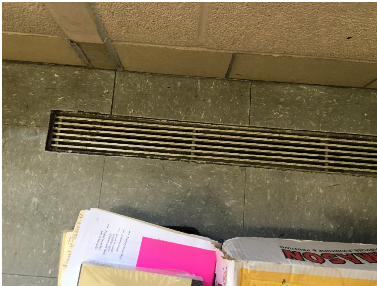
Photograph 2: Typical plenum vent in floor, Burncoat room A6
