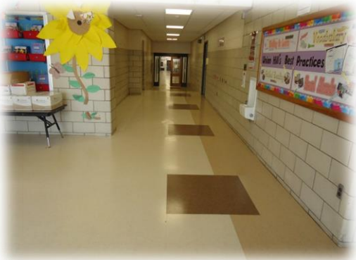
Front entrance flooring renovation
