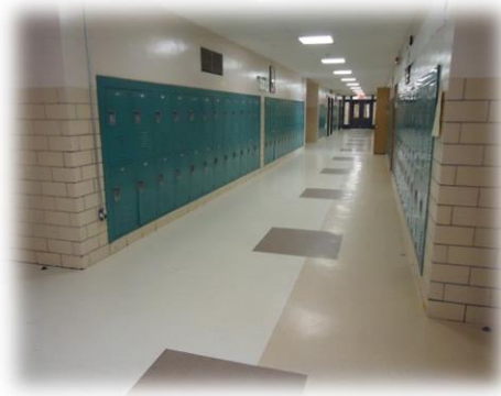
New lockers and flooring
