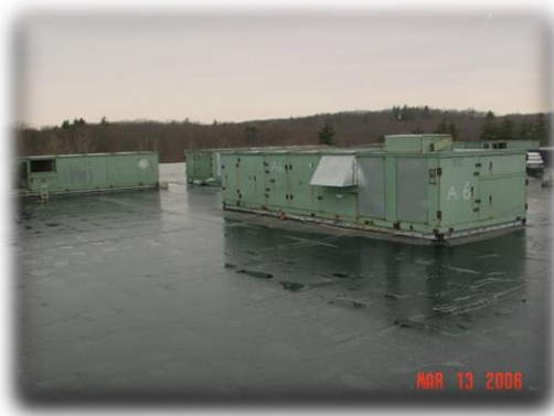
South High Old Rooftop Units
