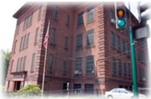
GRAFTON STREET SCHOOL (BUILDING #1) 311 Grafton Street
