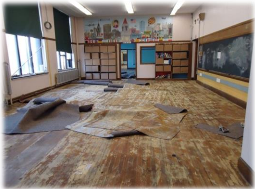
Classroom during renovation
