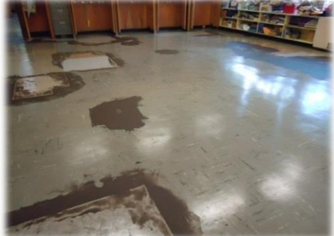
Flooring before renovation
