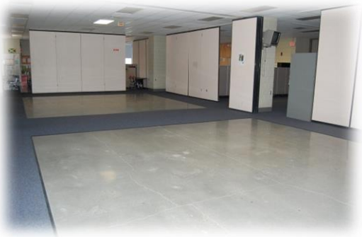
Refurbished floor and new carpet
