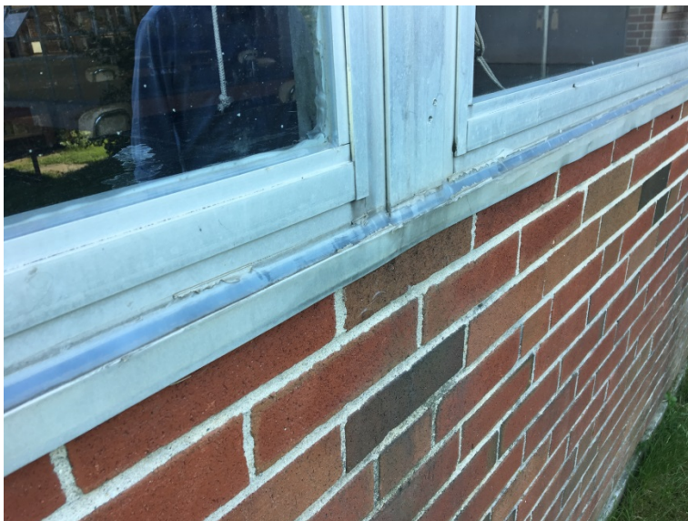
Photograph 6: Area of formerly disturbed caulk on ground floor north face of 400s wing.
