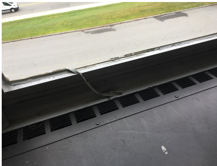
Photograph 4: Damaged caulk, Room 210
