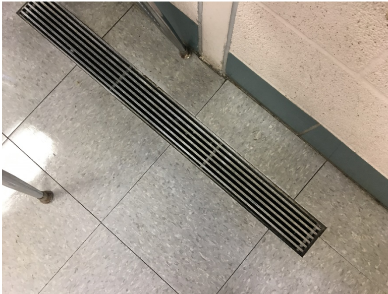
Photograph 2: Typical plenum vent, Room C19
