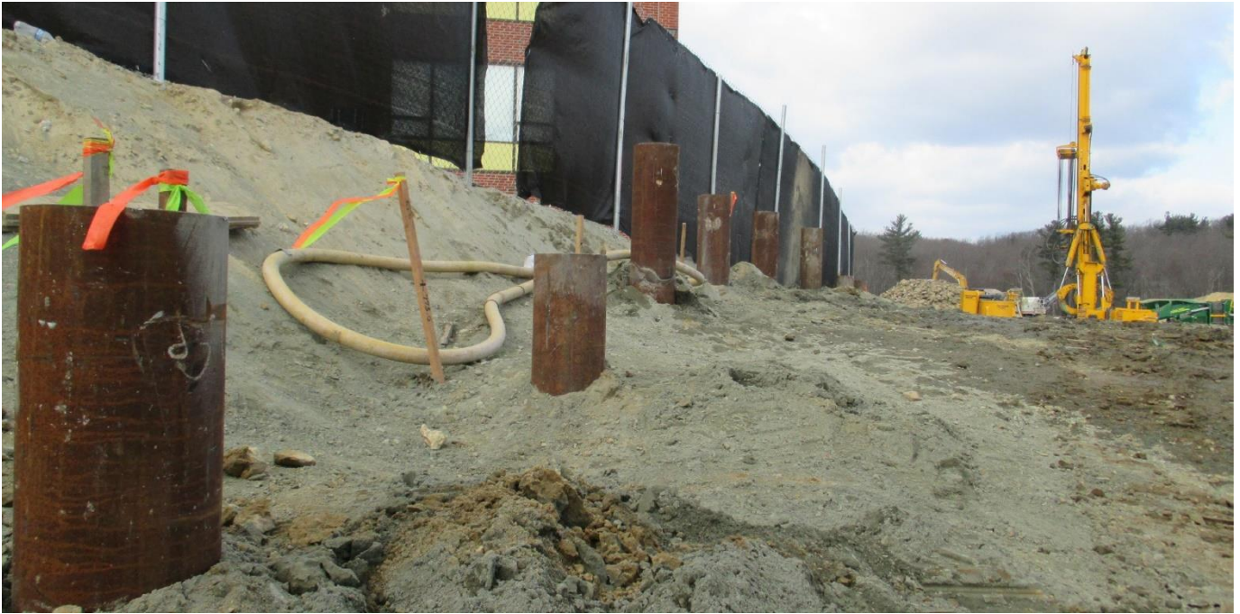
5. Piles installed for SOE system
