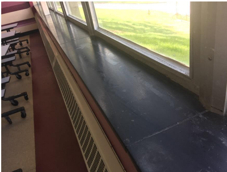
Photograph 2: Typical windowsill, cafeteria
