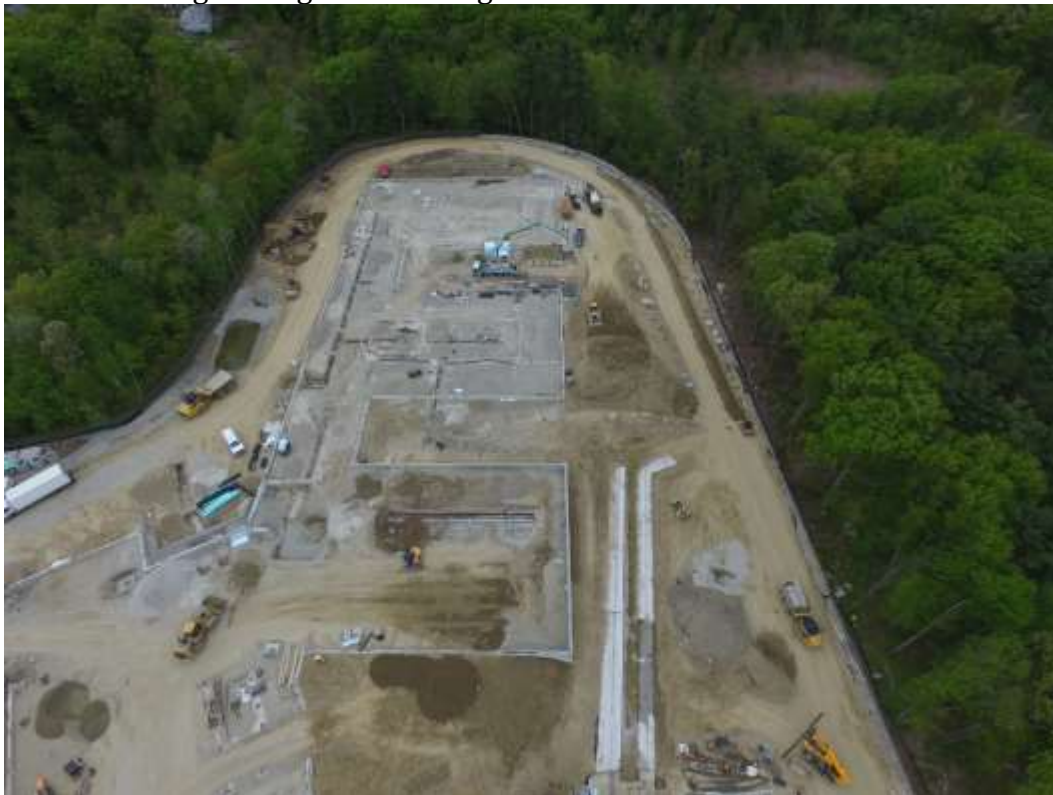
6. Progress in A building from above
