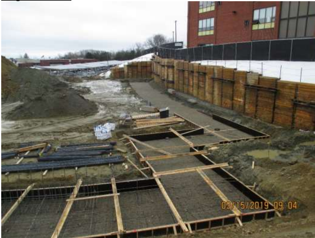
1. Prep and forms for foundation wall footings
