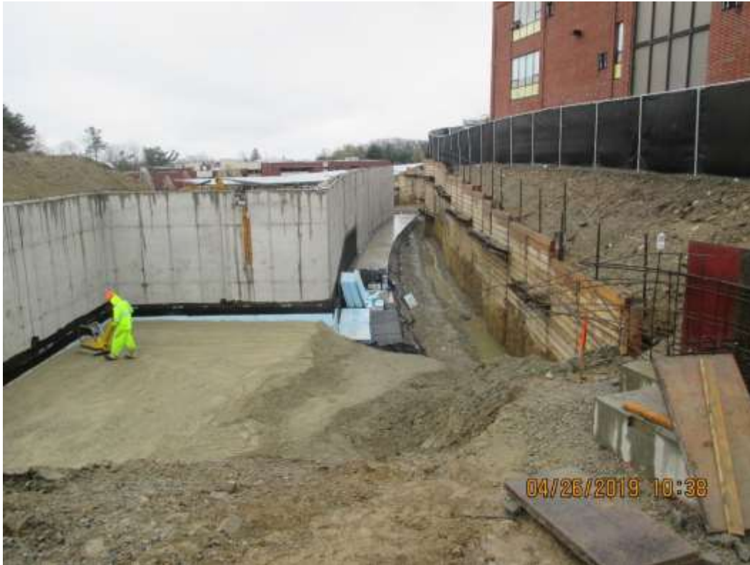
3. Back fill between foundation wall and SOE
