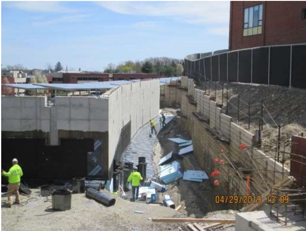
4. Waterproofing at foundation wall and footing
