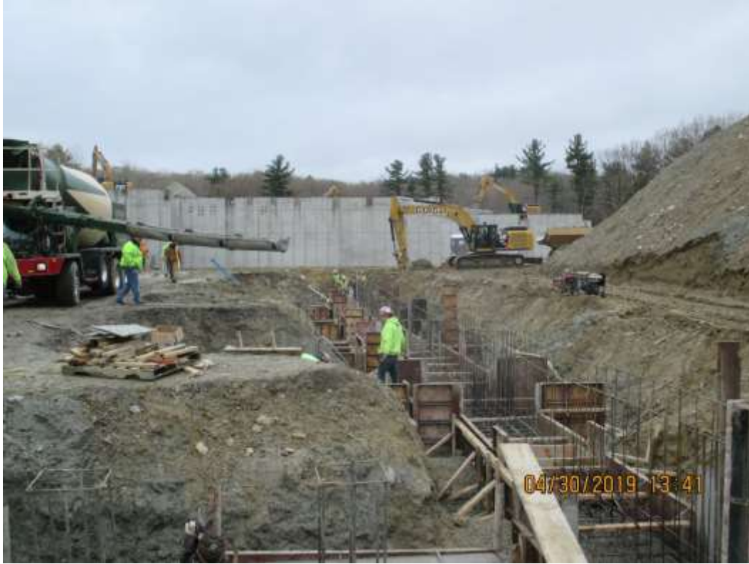
5. Pouring footing in B building
