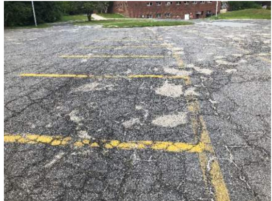
Picture 3: Pavement Deterioration Upper Parking Lot
