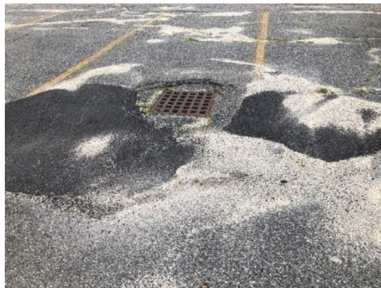
Picture 6: Pavement Deterioration East Parking Lot
