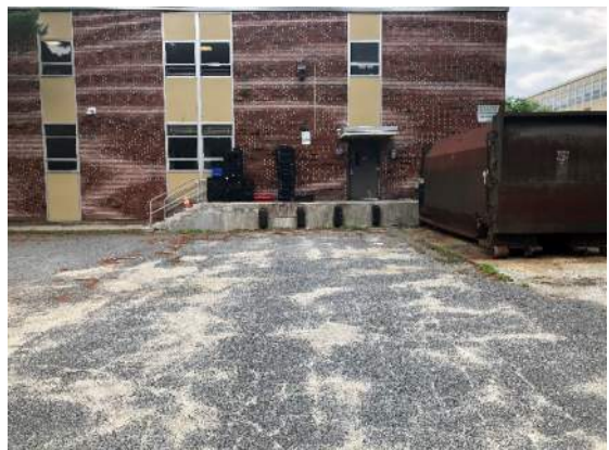
Picture 4: Pavement Deterioration Service / Loading Area
