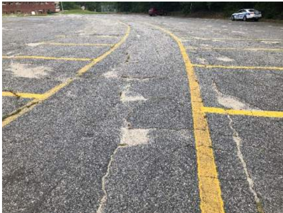
Picture 1: Pavement Deterioration Upper Parking Lot
