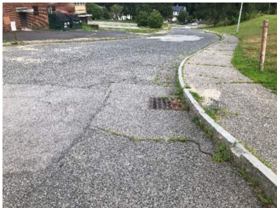
Picture 2: Pavement Deterioration East Access Drive
