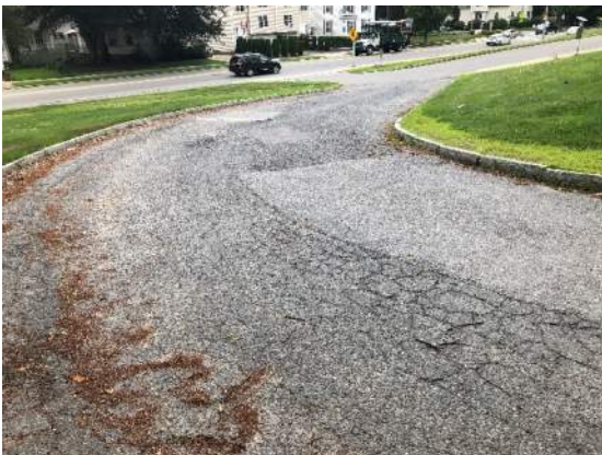
Picture 5: Pavement Deterioration Service Area Access Drive
