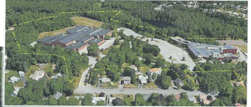
EXISTING AERIAL VIEW FROM SOUTH
