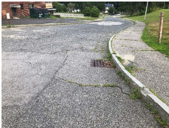
Picture 2: Pavement Deterioration East Access Drive
