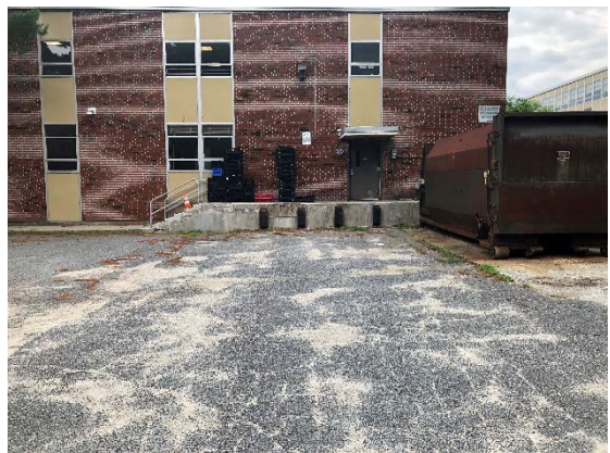
Picture 4: Pavement Deterioration Service / Loading Area
