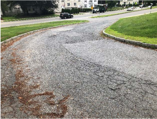
Picture 5: Pavement Deterioration Service Area Access Drive
