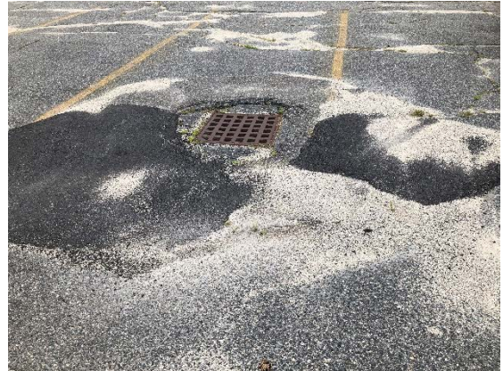
Picture 6: Pavement Deterioration East Parking Lot
