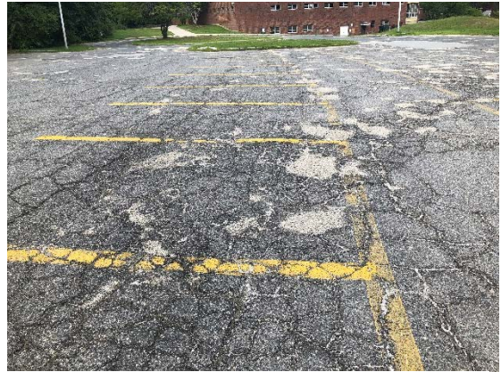
Picture 3: Pavement Deterioration Upper Parking Lot
