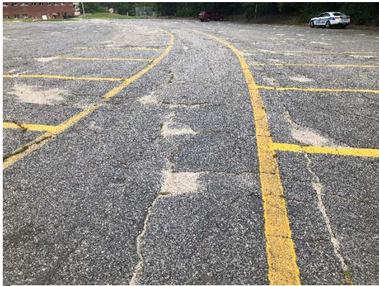
Picture 1: Pavement Deterioration Upper Parking Lot
