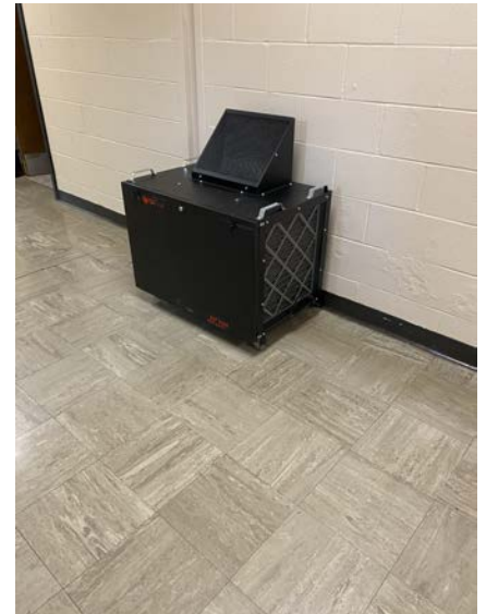
Needlepoint Bipolar Ionization Units Throughout Building
