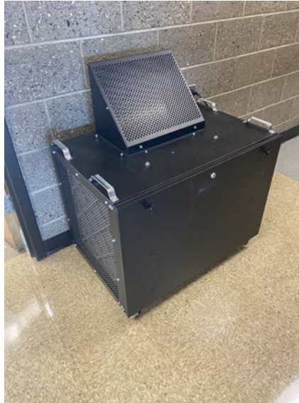
Needlepoint Bipolar Ionization Units Throughout Building
